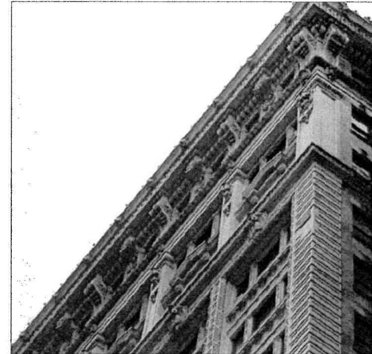
The façade is clad in ornate terra cotta detailed with Classical ornament derived from the French Renaissance style, as shown here in two current photographs.
